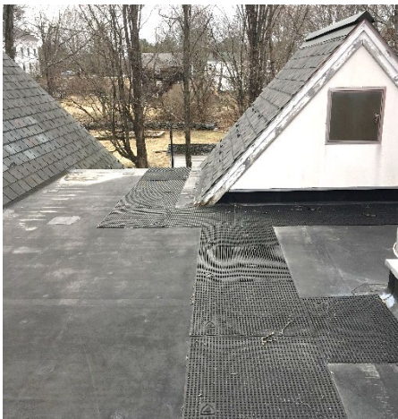
Flat roof at new addition.
