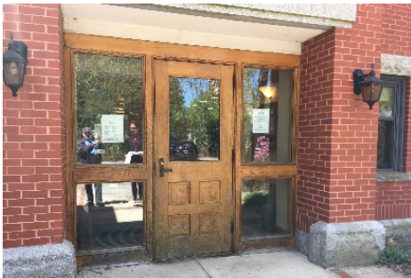
East Main Entry Door
