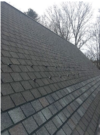
Four courses of shingles which replaced venting on roof of addition.
