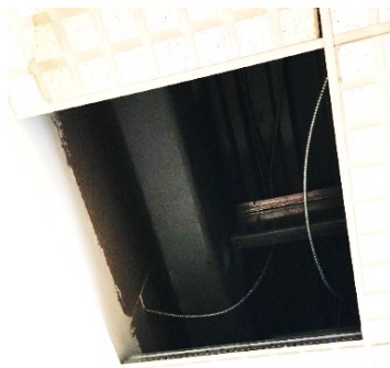
View of Beams and Decking in Addition
