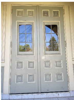
North Egress Doors
