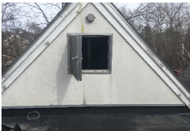
Gabled areas over main entrances in addition.
